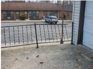
Photo C: A broken banister that has become detached from the structure and is no longer is safe for tenants to use. This is a health and safety issue that would be classified as a program violation.
