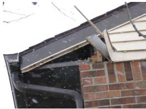
Photo B: Hole in the side/roof of the apartment building due to missing siding. The hole is large enough for animals to enter the attic area of the structure. Tenants reported that birds were living in between the ceiling and the roof of the building. This deficiency would be classified as a program violation.
