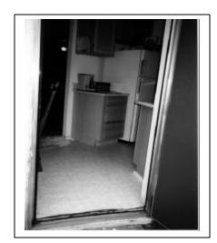
Although three inspection reports had been completed, none indicated any problems with the construction work. Our inspection of the home disclosed that the vinyl flooring was not tacked down, door molding was not installed at the kitchen entrance, and the flooring for the front porch was higher than the front door stoop. These defects are safety hazards that should be corrected. The CDM told us he was unaware of these defects, and for this reason they were not listed on the inspection report.
