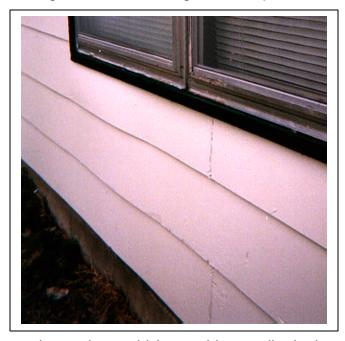
the first inspection, he reported, "there were questions on replacing the masonite, and the contractor needs change out some masonite and window sills." His final inspection in November 1999 showed "all work is completed, changes were made as requested, and the work is satisfactory." Our inspection of the home disclosed the masonite siding was buckling in three places, two of which were under windows. The CDM, who was with us on
