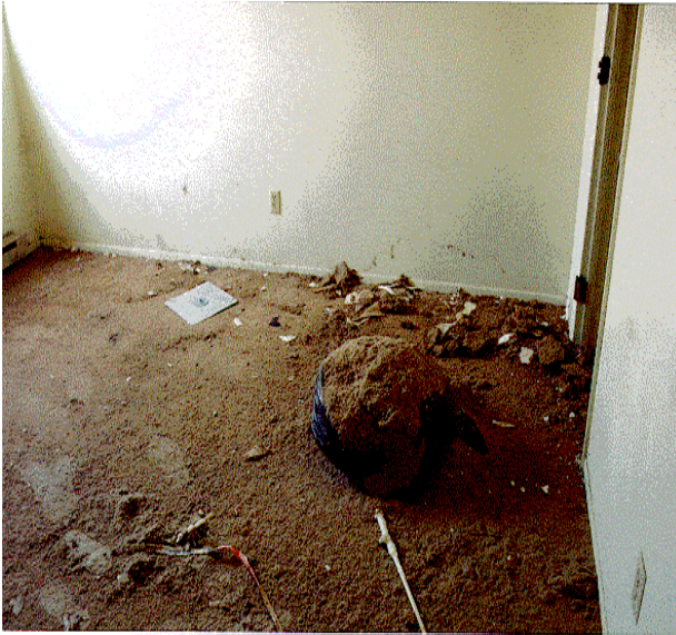
Insulation and debris on apartment floor from collapsed ceiling (due to leaking roof)
