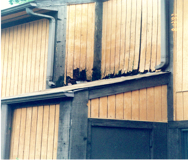
Rotting exterior siding
