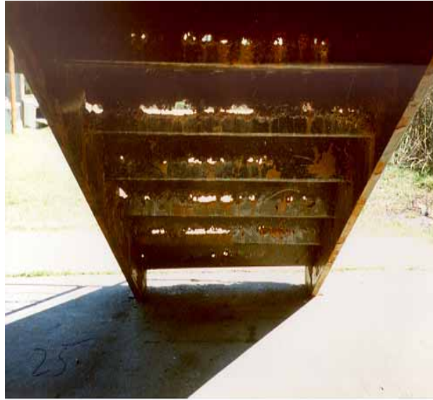
Severely rusted stairs
