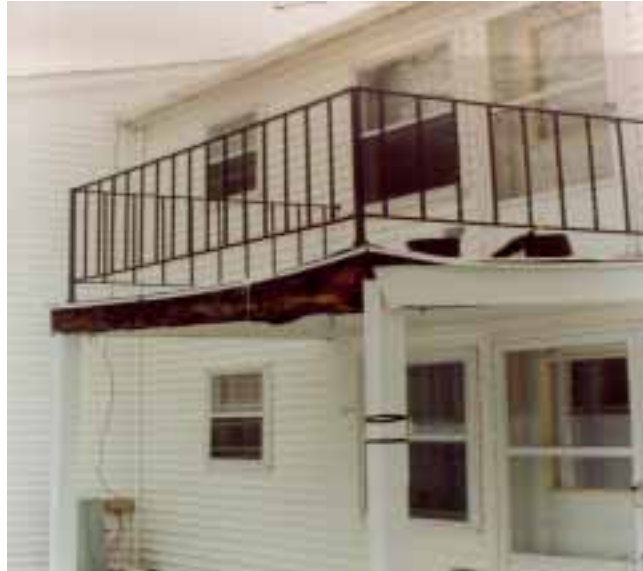
Balcony on the verge of collapse
