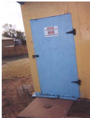
No. 5 Poorly constructed wooden storage shed with exposed easily removable hinges on the door, potentially allowing easy access to a variety of dangerous poisons stored inside.
