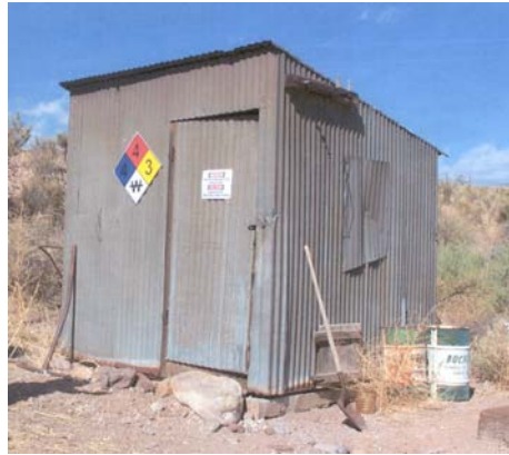
No. 6 A shed containing Fumitoxin and M-44 cyanide capsules, made of thin metal with an ill-fitting door.
